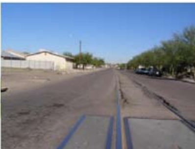
Railroad tracks pass through the middle of the neighborhood.
