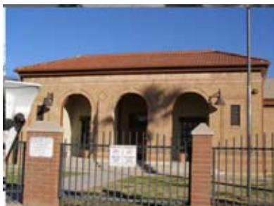
Historic Property 11: Dunbar Paul Lawrence Elementary School (Phoenix Elementary School District.)
