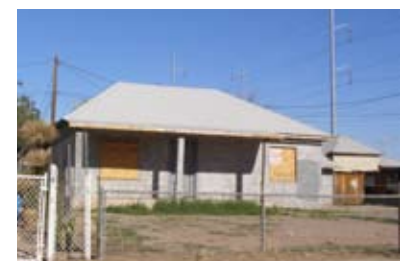
Single-family housing conditions varied but many were in poor state.
